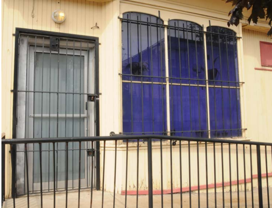
Locked emergency access to Gosnell's clinic
